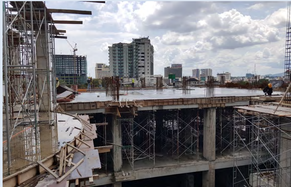
Figure 2. Suspended Slab in Progress
