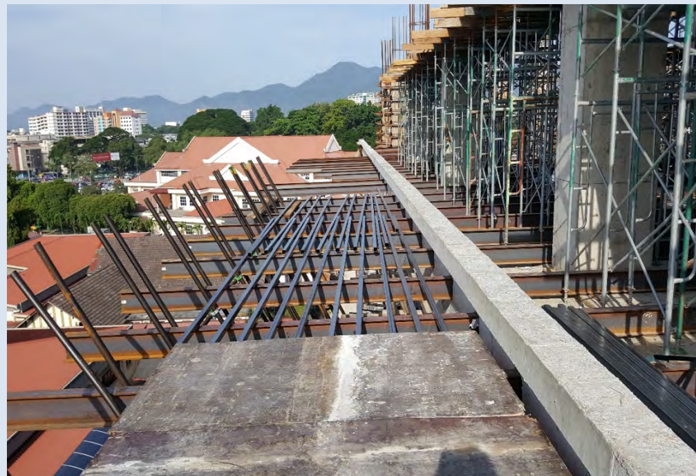
Figure 3. Elevated Temporary Platform
